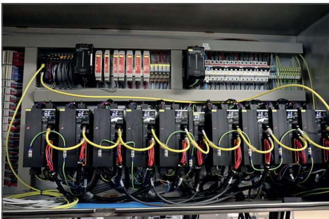
*The basis of the retrofit solution is the Sysmac automation platform in addition to OMRON's 1S drives with continuous integration from the NX/NJ machine controller to the software.*
