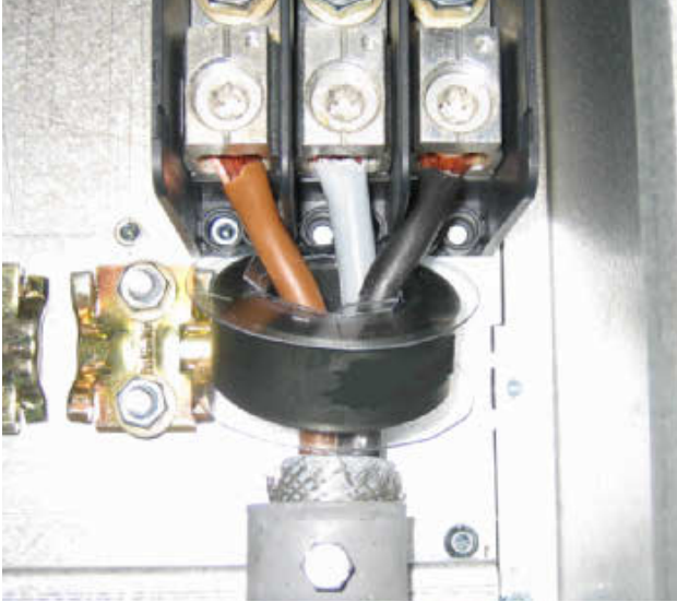
Fig. 55 Ferrite core mounted on the motor cables
