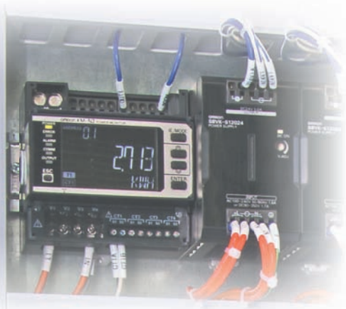
DIN Rail Installation Type KM-N2
